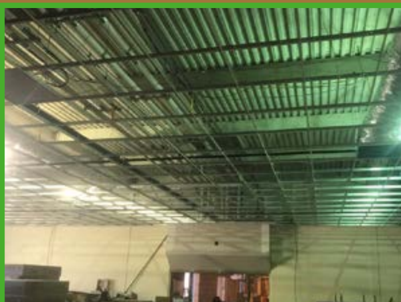
CEILING GRID INSTALLATION IN CAFETERIA
