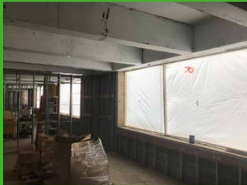
PERIMETER WALL FRAMING AND WINDOW PLASTIC SHEETING
