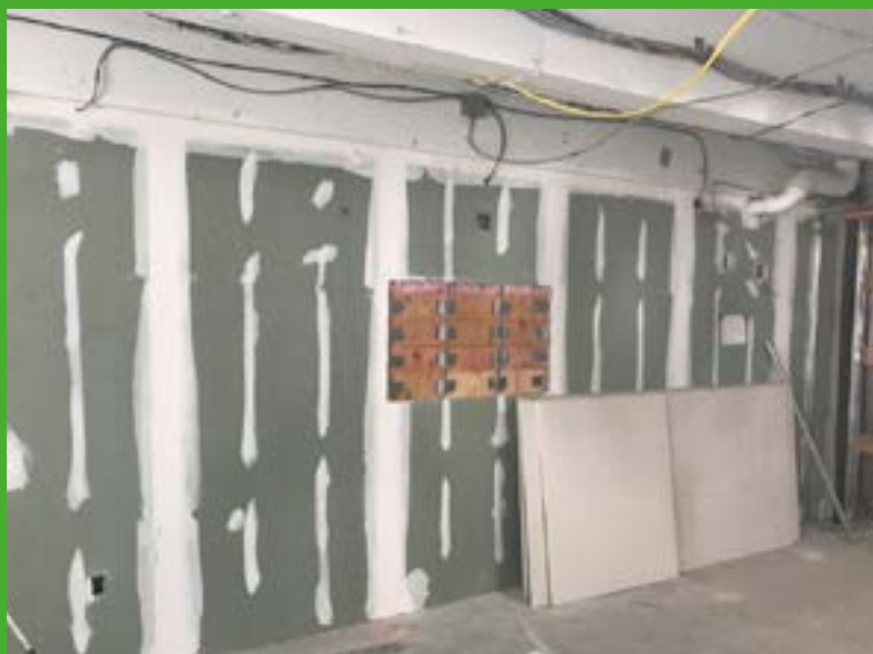
SMARTBOARD SUPPORT BLOCKING INSTALLED (TYP.)
